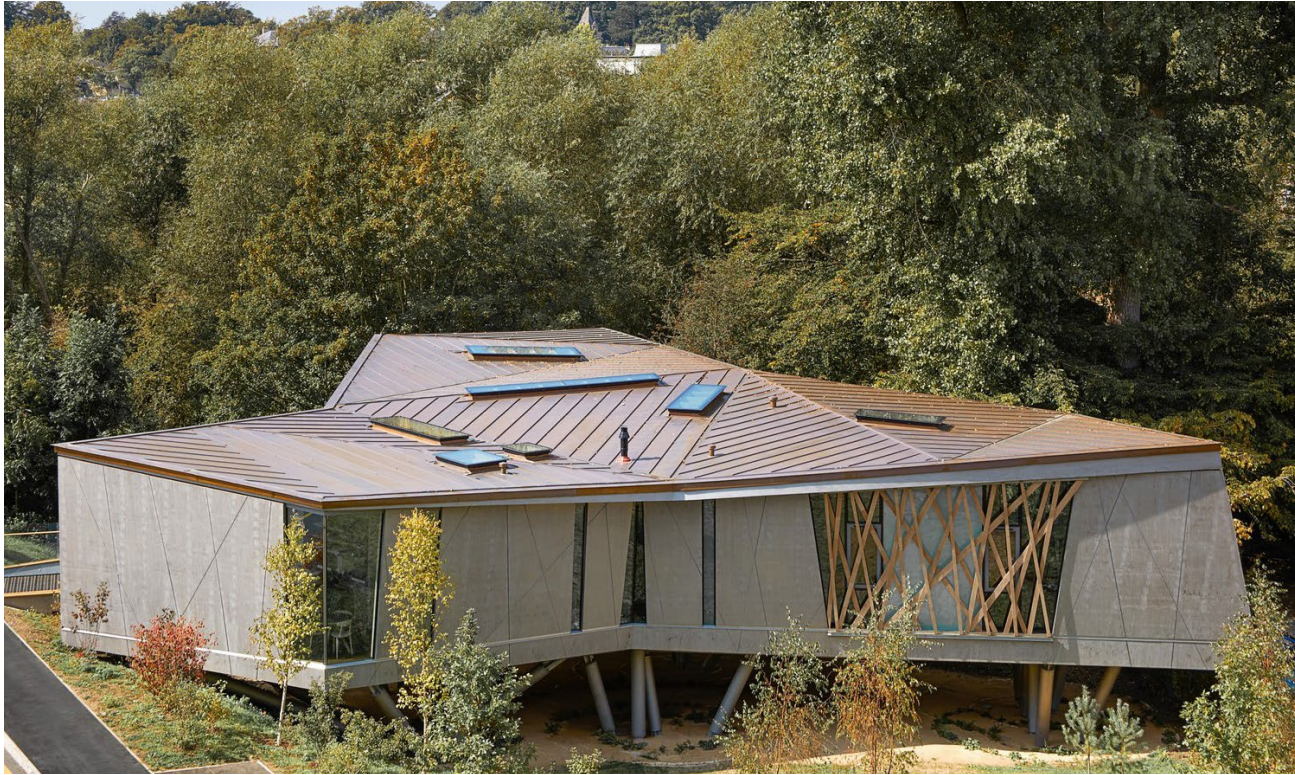
Figure 12.35 View from Northeast
