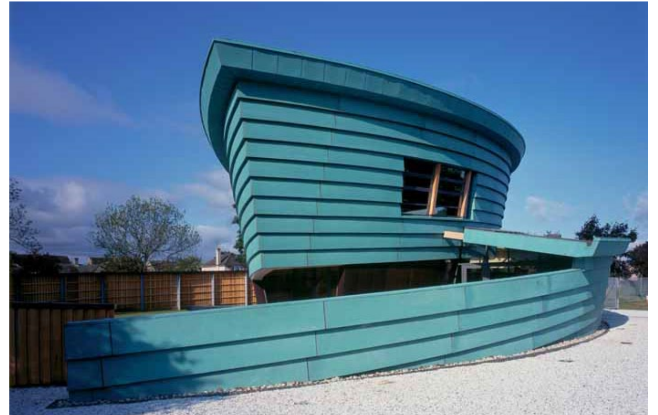
Figure 4.51 View From Northeast
