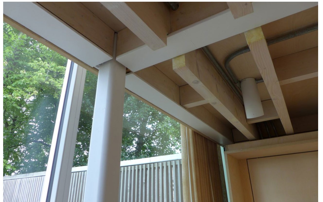
Figure 13.15 Interior Materiality - Limed Oak for floors - White Stained Pine for ceilings - Blond Finnish Birch for walls - White painted steel columns
