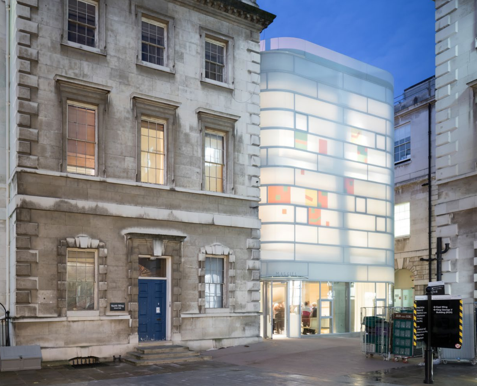
Figure 16.2 Maggie's Barts, Courtyard Entrance
