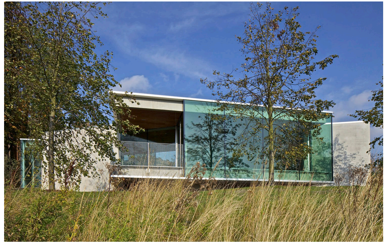
Figure 2.19 View from the parking lot up to the Kitchen area
